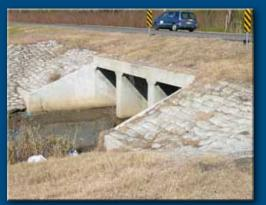
Burlap Concrete Revetment - Rip Rap can be used to install running bond retaining walls and erosion control around culverts.
